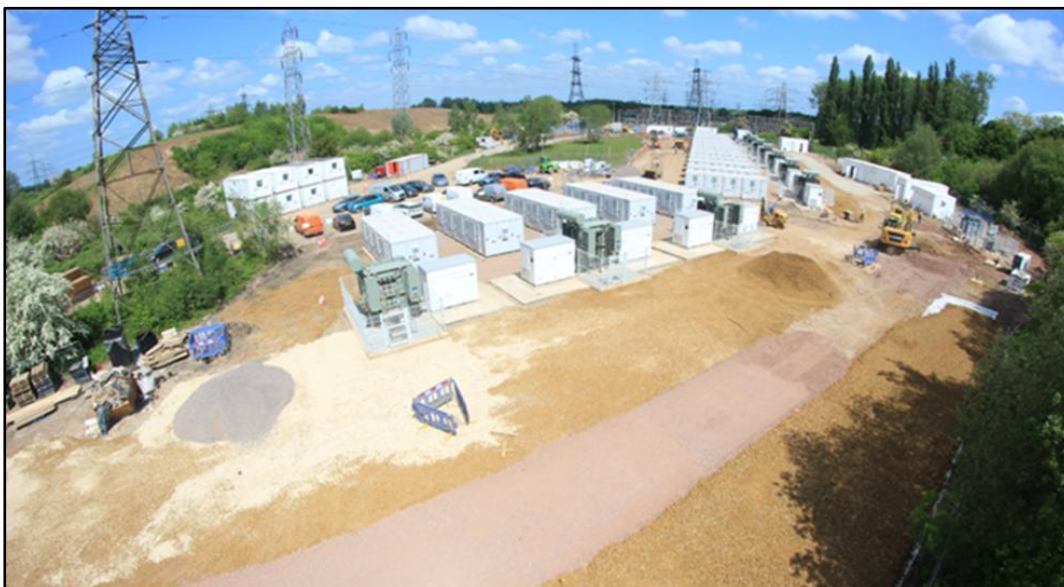
Plate 3.10: Example of the construction of BESS Compound
