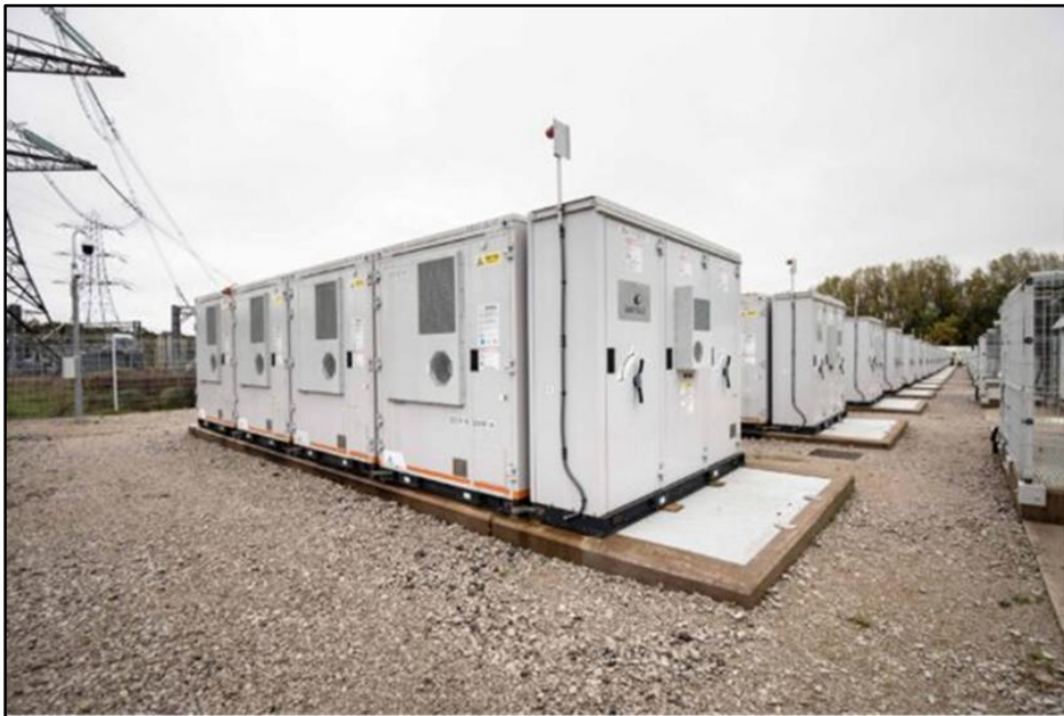
Plate 3.10: Example of the construction of BESS Compound
