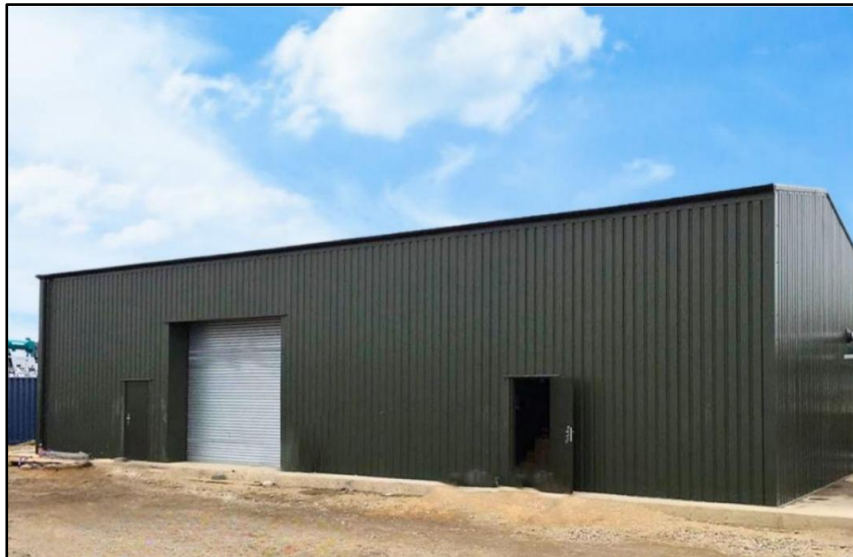
Plate 3.11: Example of a Collector Compound
